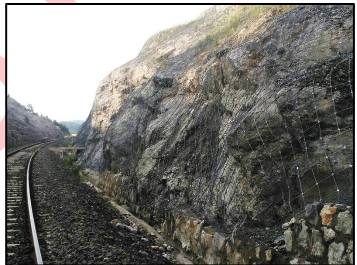
Figure 5 After installation finished
