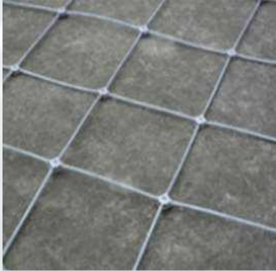
Rhomboidal cable net
