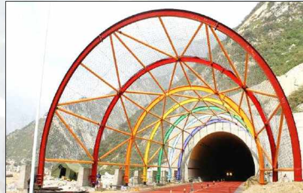
Tunnel portals along Highways
